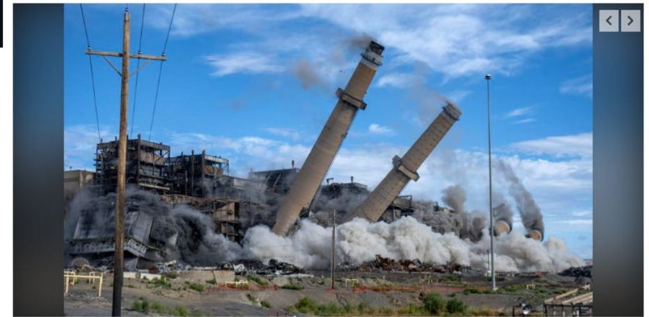
Explosives take down the four smokestacks at the San Juan Generating Station, west of Farmington, on Saturday. Eddie Moore/Journal
